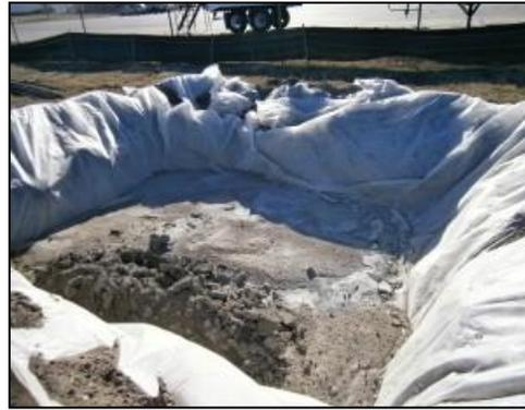
Plate 3-1 Typical concrete wash out areas
